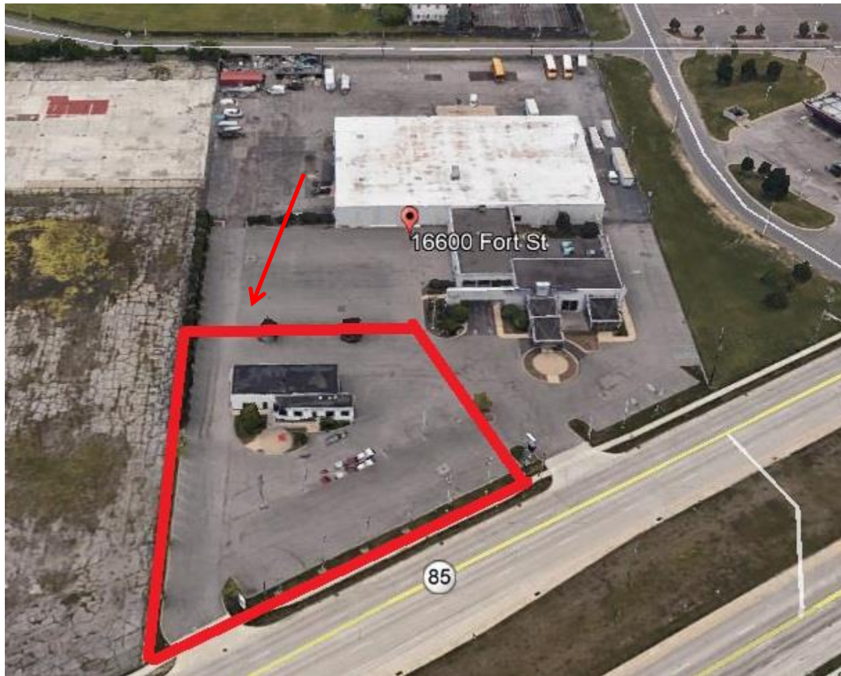
Figure 1. Aerial Photograph of Subject Site
